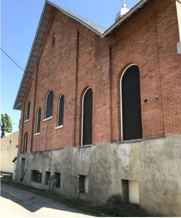
Above: view of rear elevation (west)
