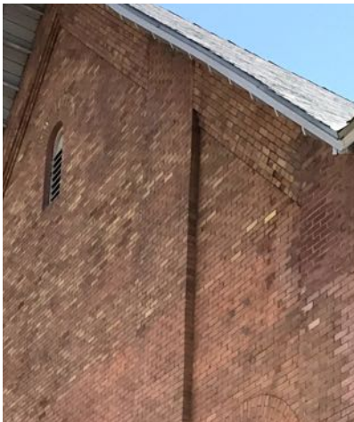
Brick repair on the back wall showing different types of bricks used, different mortar types and joint width. This needs to be monitored as incompatible materials can cause additional damage
