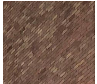
Brick repair on the back wall showing different types of bricks used, different mortar types and joint width. This needs to be monitored as incompatible materials can cause additional damage
