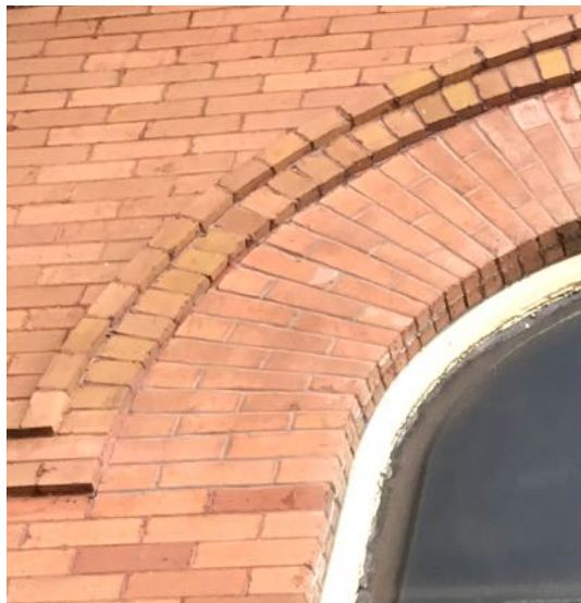
Far left: On the back wall expanding spray foam has been used to unsuccessfully fill gaps between the soffit and brick. Other gaps show activity from birds looking for nesting places in the roof.
