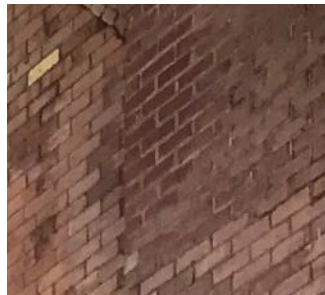
Brick repair on the back wall showing different types of bricks used, different mortar types and joint width. This needs to be monitored as incompatible materials can cause additional damage
