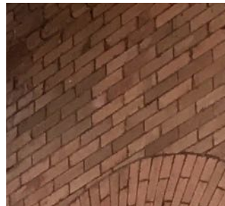
Brick repair on the back wall showing different types of bricks used, different mortar types and joint width. This needs to be monitored as incompatible materials can cause additional damage
